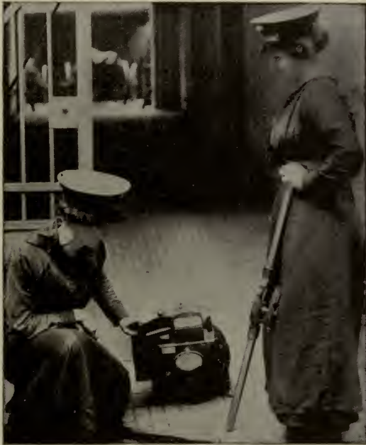
Reading the Gas Meter.
